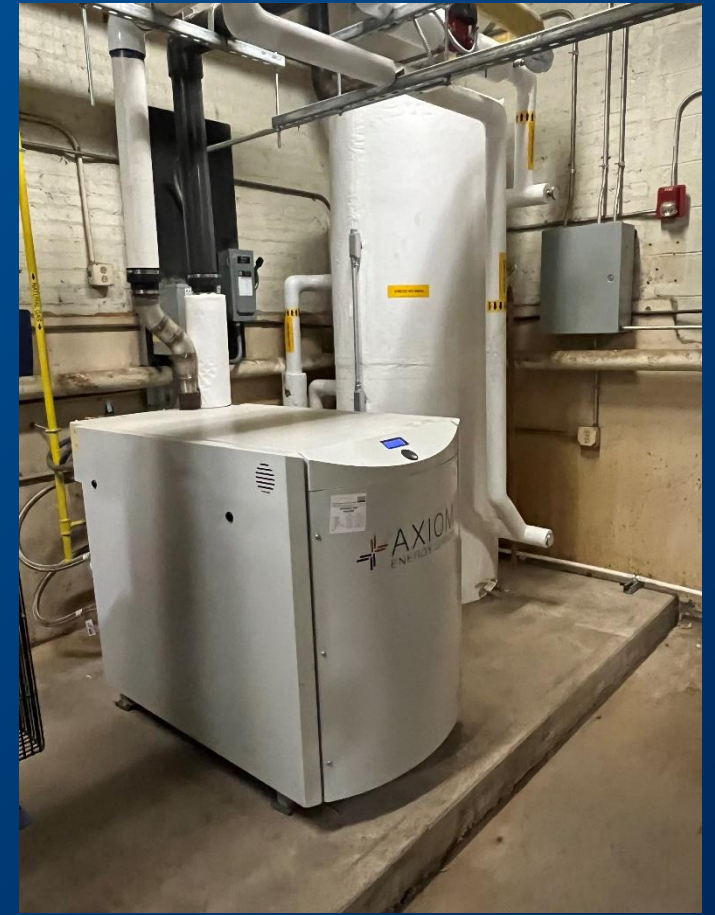
•Combined Heat & Power Generator
